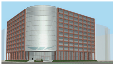
■ TSINGHUA-ROHM ELECTRONIC ENGINEERING HALL / Image
